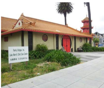
Temporary LMCC site at 7th Street
